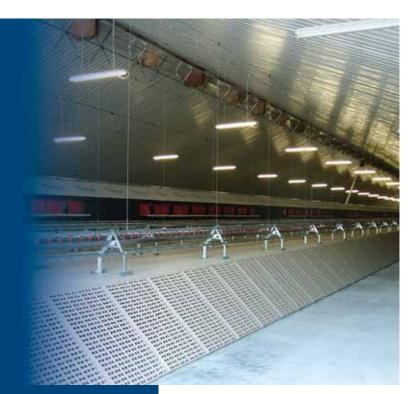
The Potters Poultry plastic slat is probably the strongest and most stable available and you will feel safe and steady when walking on them. We use a very simple galvanised steel and plastic structure beneath the slats for support. The legs are fully adjustable and can cope with variable floor levels.
